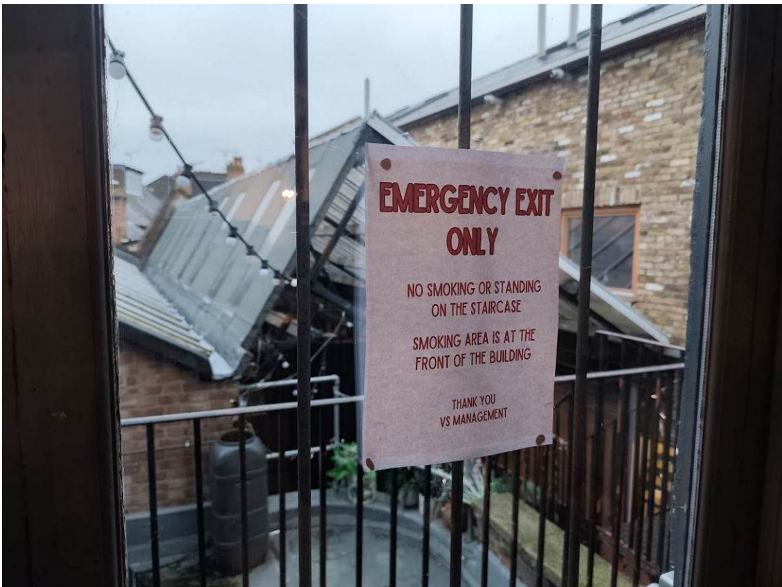
Figure 8: Signage at the function room emergency exit, note covered courtyard area in the background
